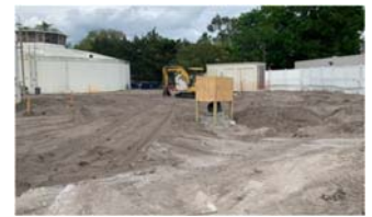
Pictured: Demolition of the existing Howell Park Water Treatment Plant.
